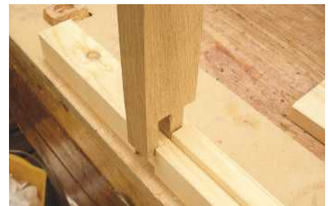
▲ Pic.15 Mortise & tenons joint the sashes, only the joint between the rails and stiles differing
